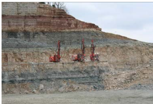
left: Amrize Cement Quarry
